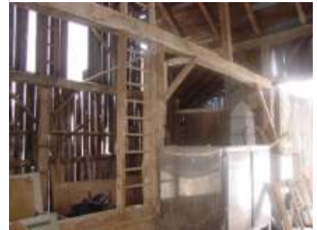
The Swing Beam creates this loft and an open space without posts below
