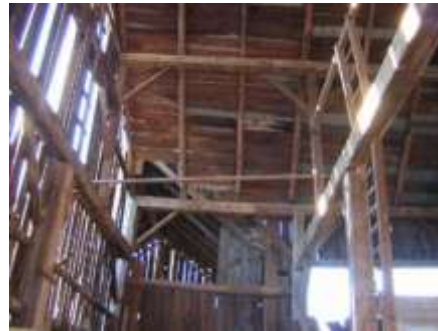
The Swing Beam creates this loft and an open space without posts below
