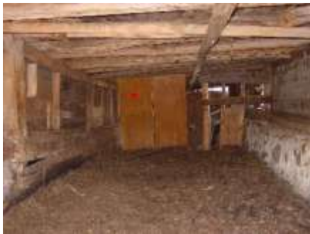
The Swing Beam creates this loft and an open space without posts below
