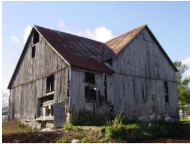
Rear- Cross Gable
