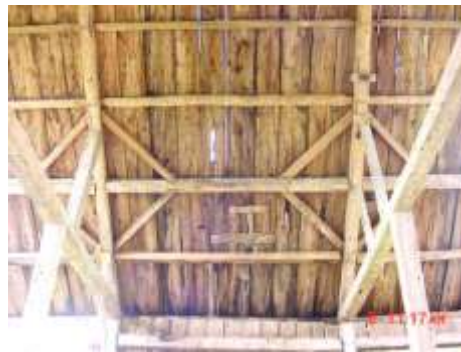
diamond wind brace & hewing detail
