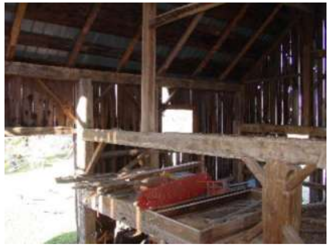
The Swing Beam creates this loft and an open space without posts below
