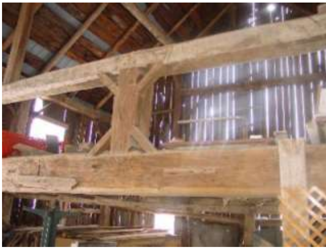
The Swing Beam creates this loft and an open space without posts below
