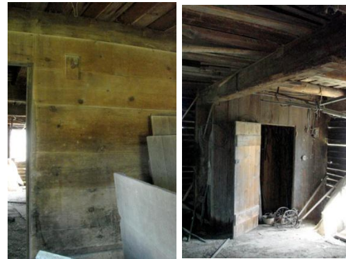
Granary Boards in the Barn
