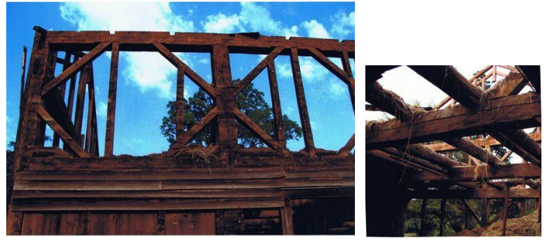
Large Hand Hewn Beams in the Barclay Barn
